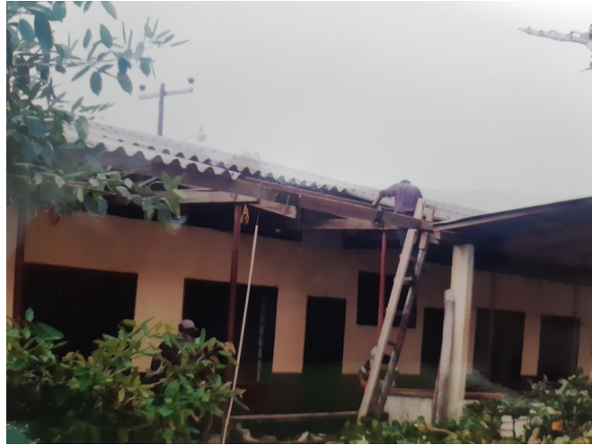
Repairing roof with 30 sheets of roofing
